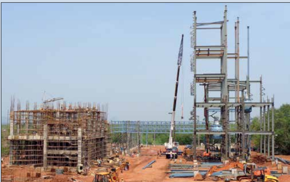
NACL Srikakulam Tehcnical Unit - Block 7 implementation in progress
